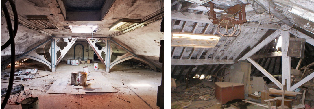
2005, Con Kehely. Central trusses on the left with end trusses on the right. The decorative inserts are modern painted plywood.
