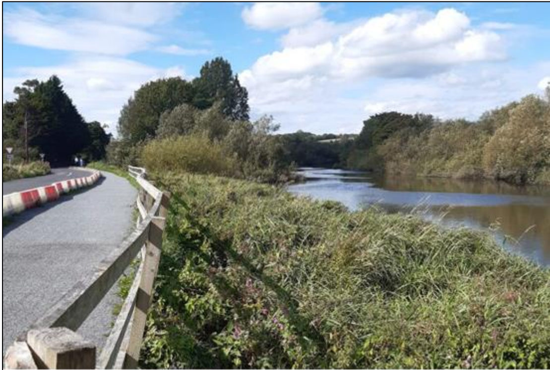
Plate 2.7 Temporary embankment constructed in footprint of burned section of boardwalk.
