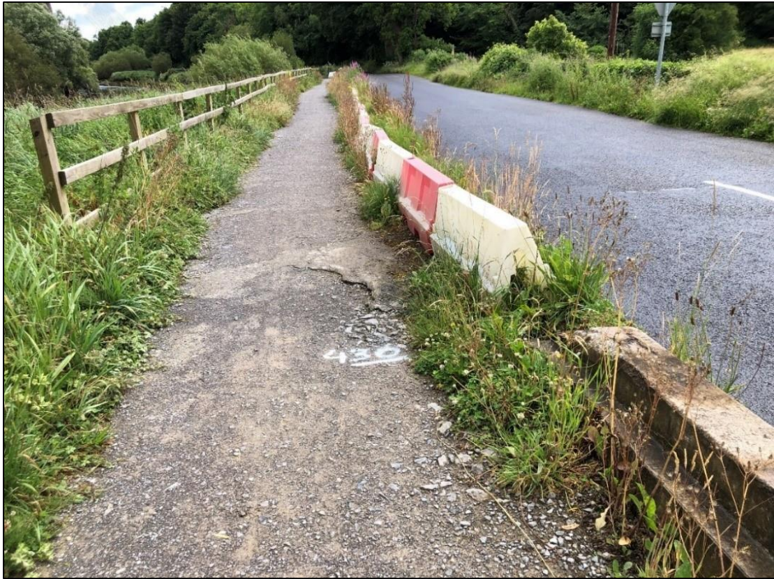
Plate 2.3 Temporary pedestrian and cycle path where boardwalk was burnt (current condition)
