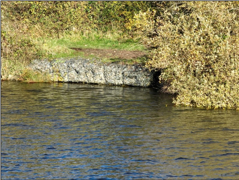
Figure 10: Existing gabions
