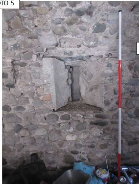
IMG_5379 Detail of window [3]. Wooden lintel and sill removed. Block wall [2] through ope.
