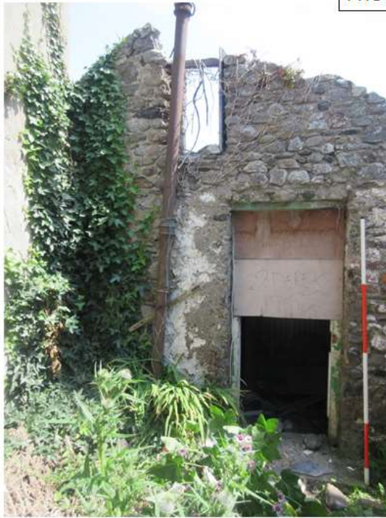
IMG_5383 SW gable end wall with Door [13] and Window [19]. Gutter downpipe seems to be a previous attachment to adjacent building [18] (to left)
