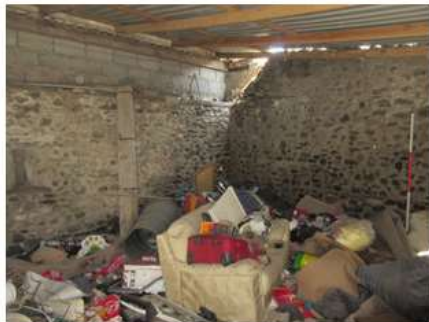
IMG_5401 E room, NE gable end remodelled for block wall and Roof [2]. Facing N
