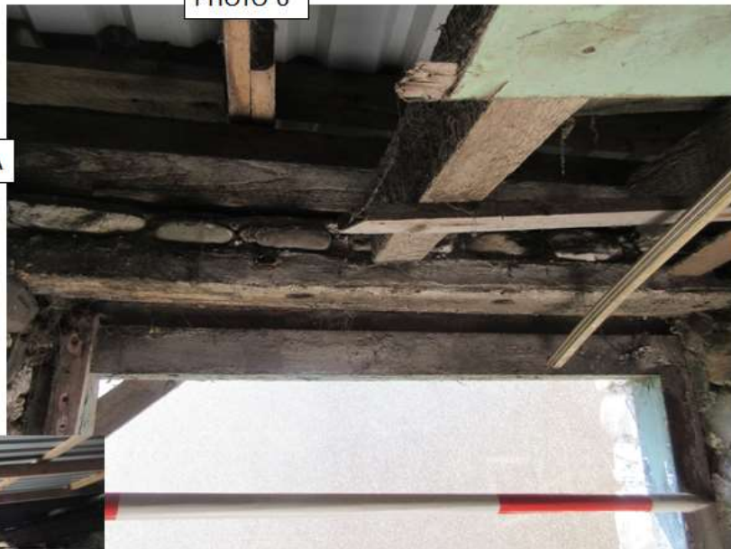
IMG_5381 Architrave of wooden horizontal Joist Treatment [20], layer of beach stones in mortar and then wooden horizontal. Over Door [10] joining with ceiling/floor [21]. Facing S
