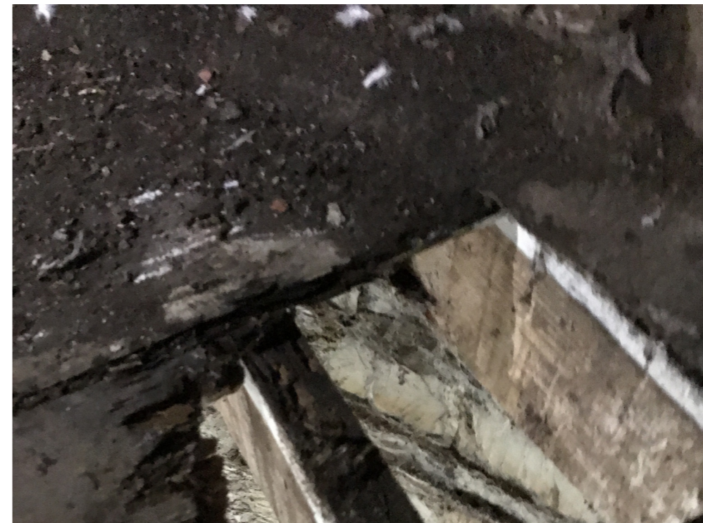
Water damaged joist ends and timber floor in the tower.
