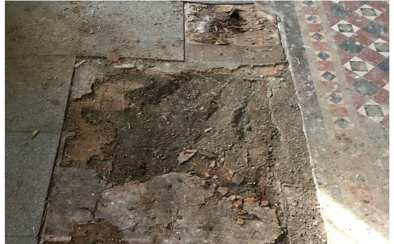
Carpet tile on plywood on earth to either side of aisle
