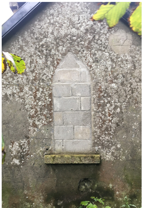
Blocked up window on north of vestry
