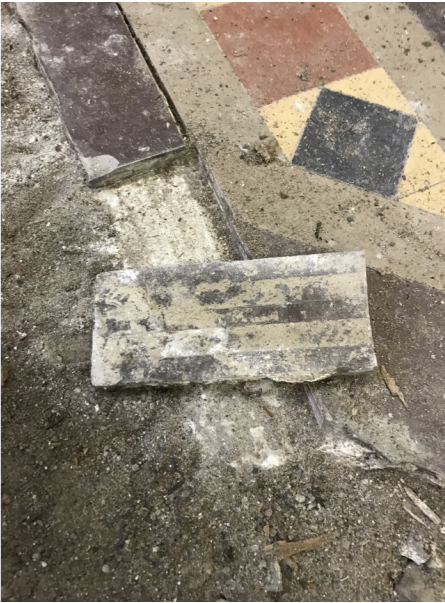
The tiles to the aisle are modern ceramic tiles.
