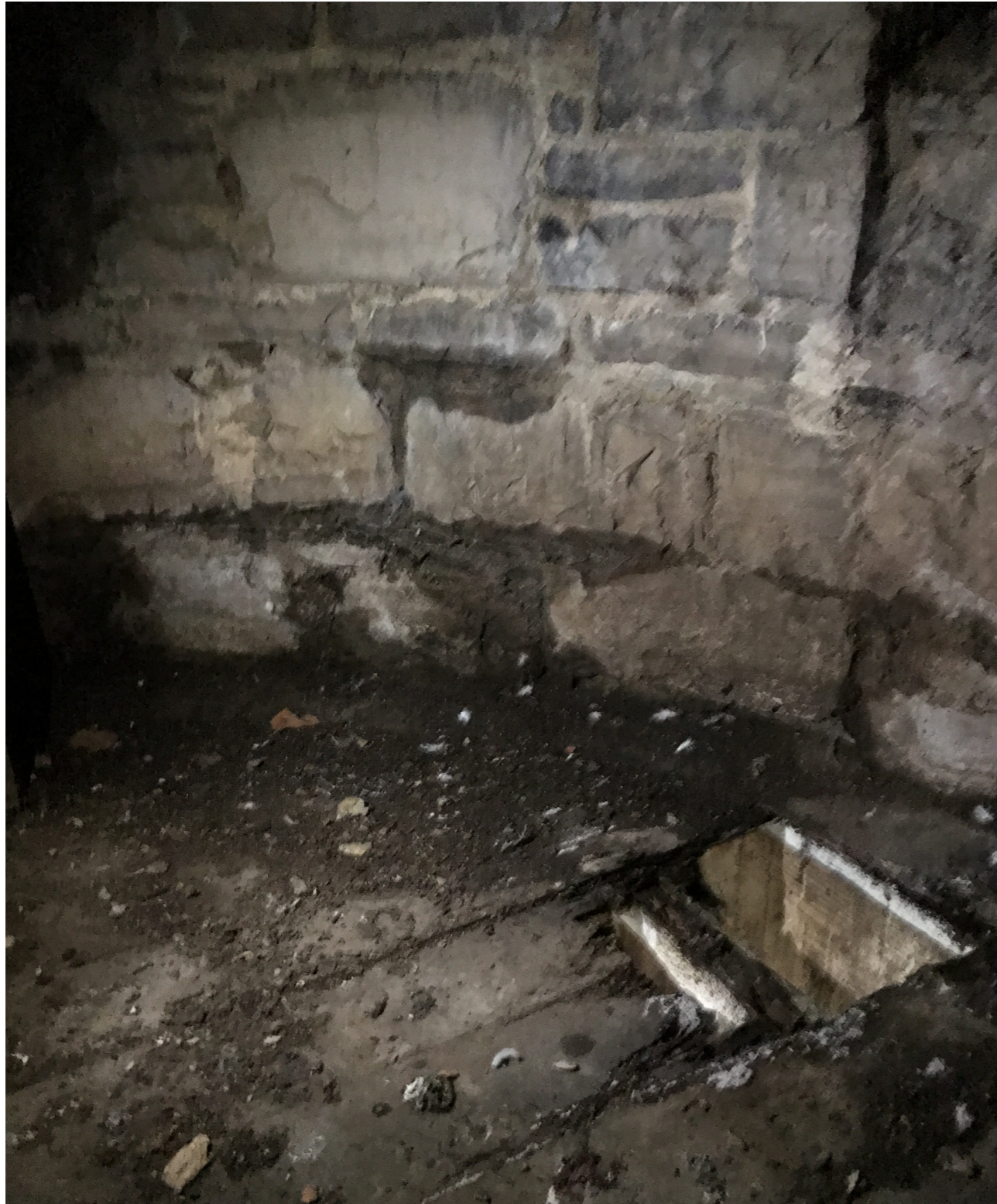
Damp patches in the wall of the tower.
