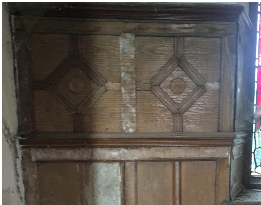
Timber veneer panelling around the chancel
