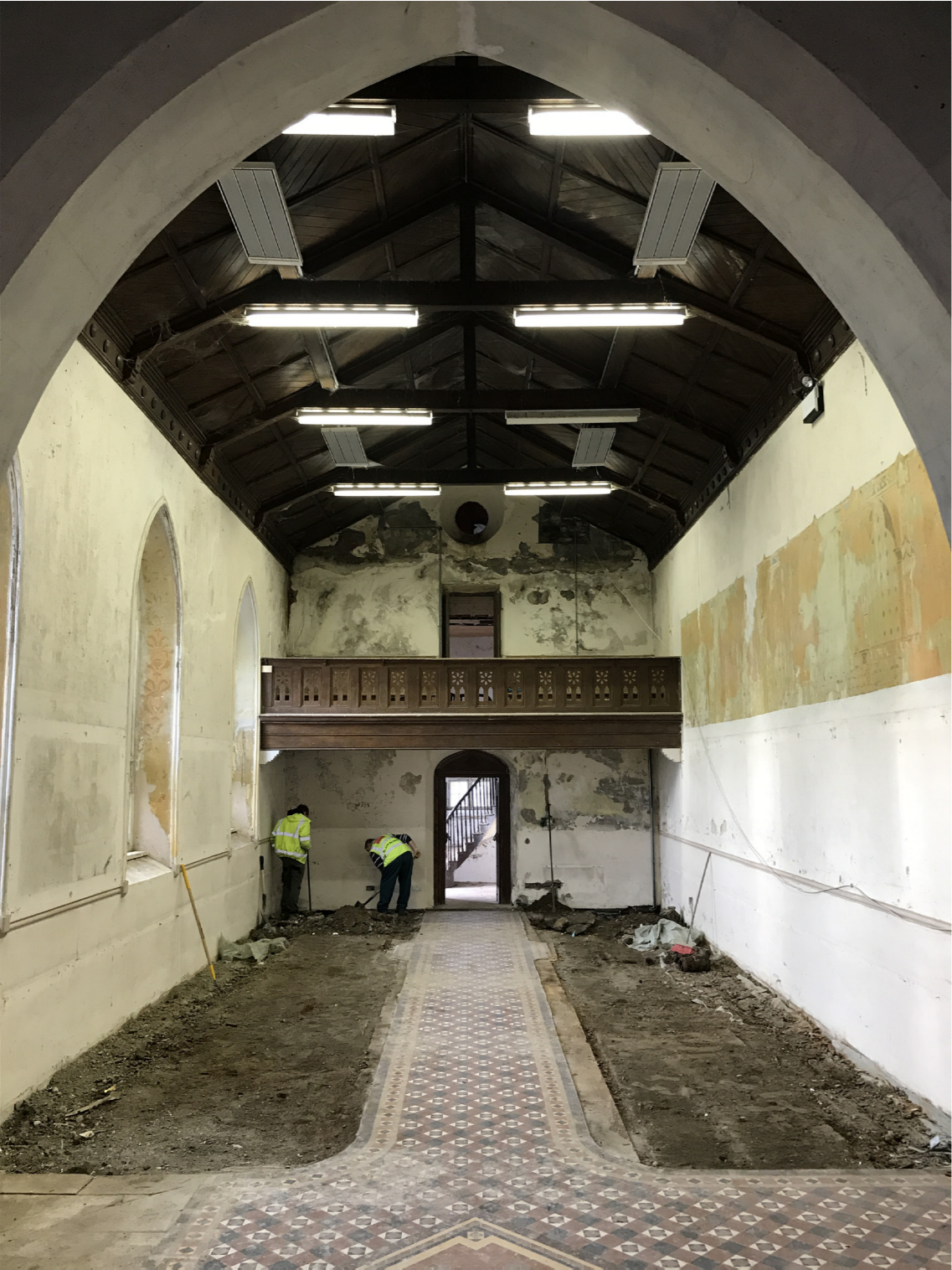
View of the nave looking west while trial holes are being dug.
