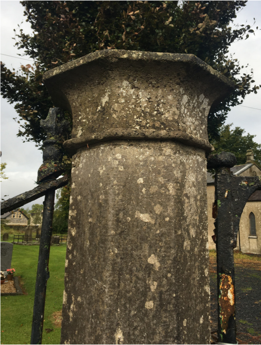
Hexagonal cut stone gate post
