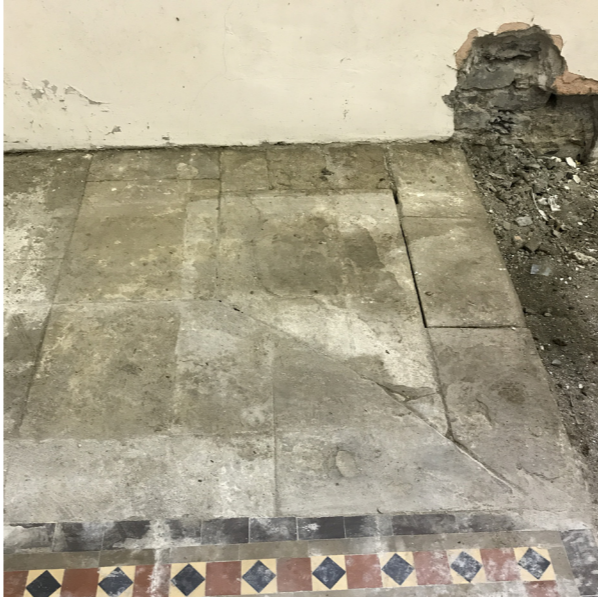
Area of stone flags laid directly on soil in the south east corner.
