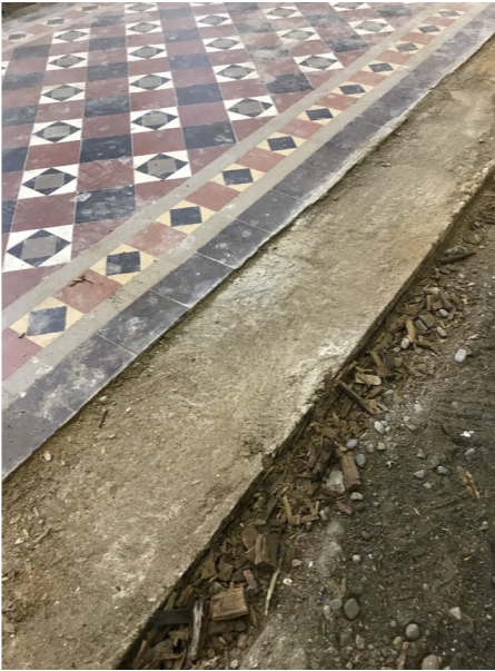
Detail of concrete base below aisle tiles
