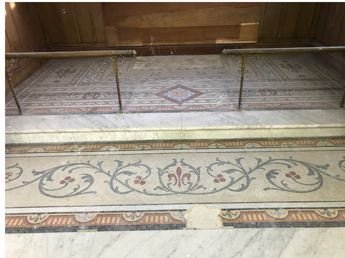
Chancel floor. Note the small area of missing tiles to the front.
