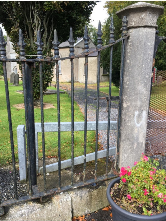
Detail of hinged opening section to the left hand side of the main gate
