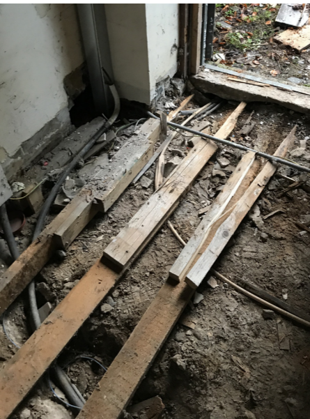
Vestry floor. Modern timber joists directly onto soil
