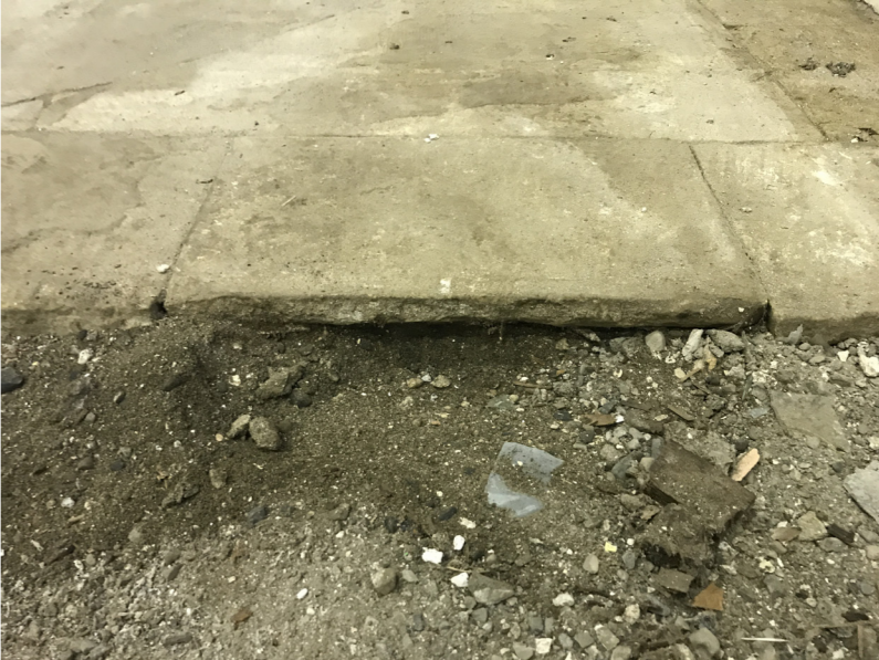
The flag stones are laid directly onto the soil below.
