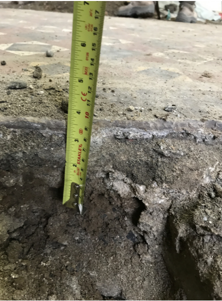
The base below the aisle tiles is approx. 75mm thick lean-mix concrete directly onto soil.
