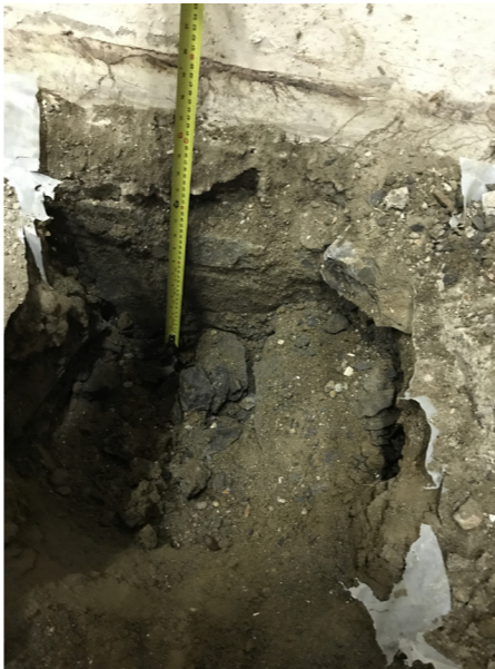
Trial hole to the edge of the nave. The external walls typically extend 500-600mm below finished floor to a stone foundation.
