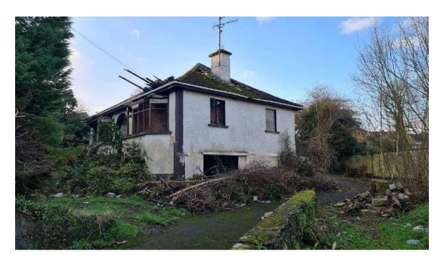
Front & north-east elevations of property with partially collapsed roof and significant overgrowth in the foreground
