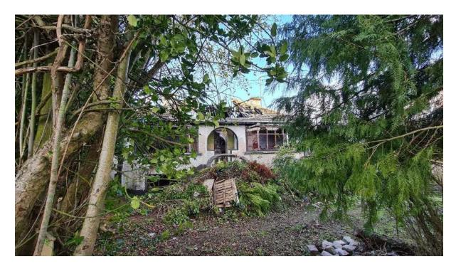
Front elevation, with partially collapsed roof and damaged windows
