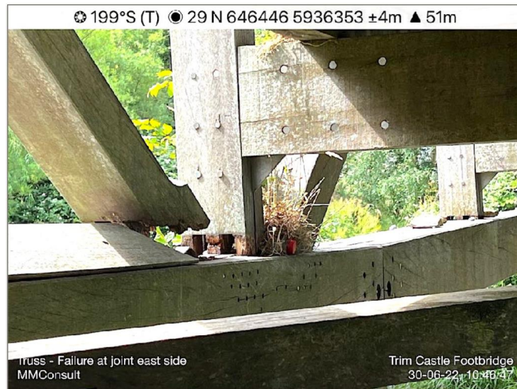
Photo P26: View of failed joint, noting unattached diagonal member and rotten ends of the members
