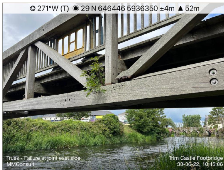
Photo P25: View of failed joint, noting unattached diagonal member and kink at splice location
