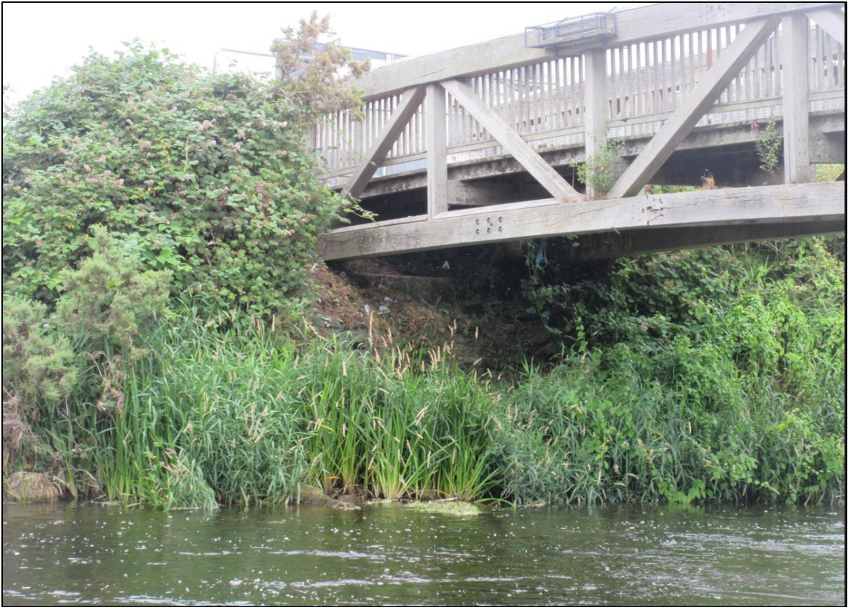
Northern abutment. Top of mass concrete block abutment may be visible.
