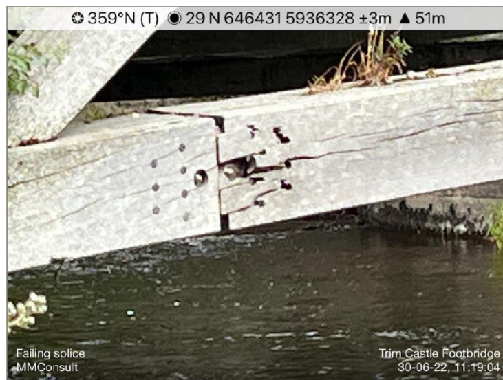
Photo P32: View of a failing splice connection to east truss at the south end
