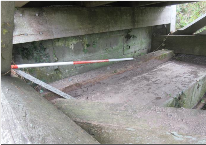
Cracking in Masking Wall on N abutment
