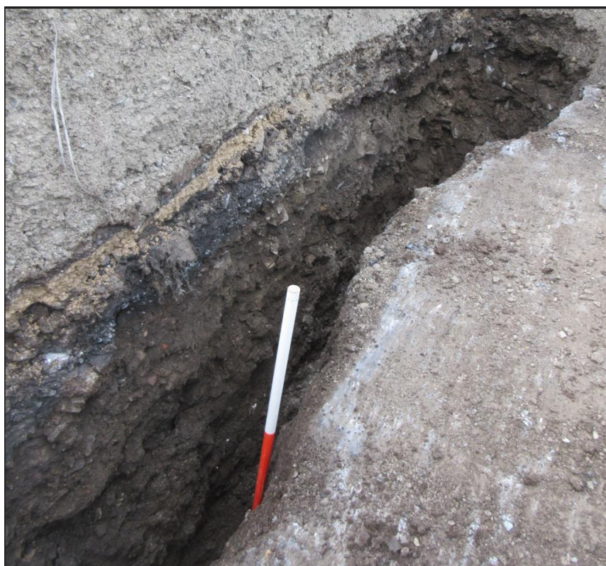
Sl.1 general section face. The abutment on right was exposed for 1.50m. The upper deposits on left are infill [12] with tip lines visible and the lower are probably the old floodplain [11]
