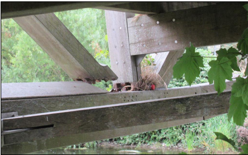
Broken joint on bridge E side
