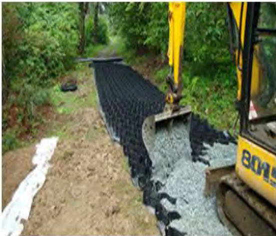
Figure 15: Proposed Geocell track design and boardwalk design where seasonal flooding is a concern
