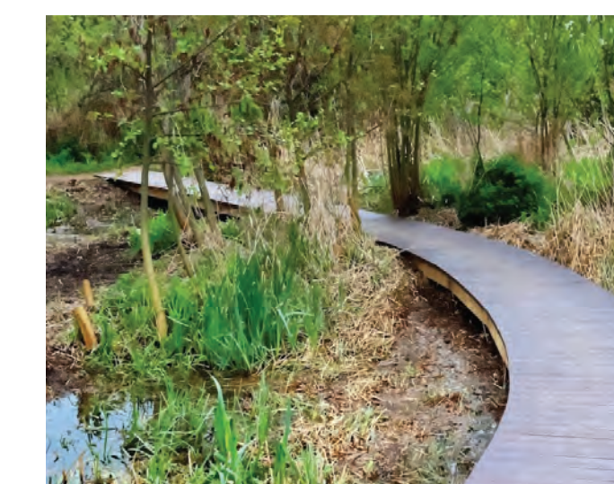
Simple boardwalk, ungraded for access, to allow for riparian zone regeneration and planting whilst allowing pedestrian access over wet spots on the trail.
